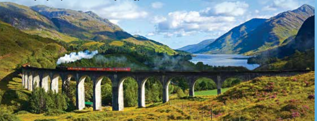
Winding through the austere Scottish Highlands, the 21-arch Glenfinnan Viaduct frames Loch Shiel, where steep slopes reflect into the loch’s sparkling fresh water.
